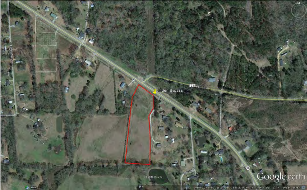
Linden Bypass DMS Site Aerial Photo
